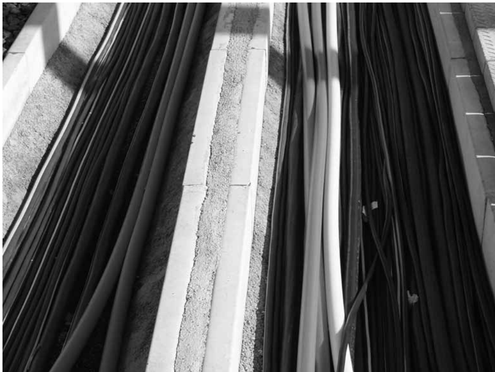
Figure 15.10 Cables between substation equipment and the control house in a hybrid substation.
